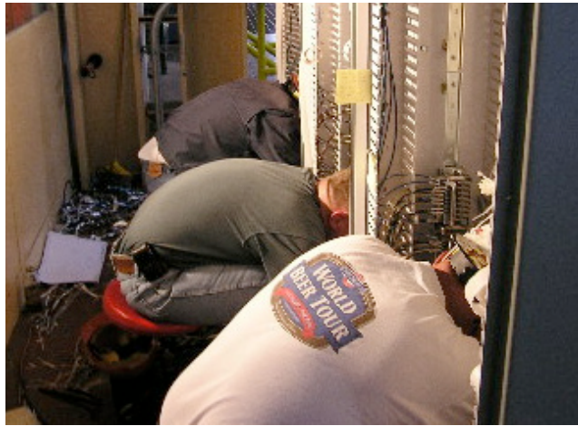
Planning and coordination paid off with only 6 cables requiring spicing.
